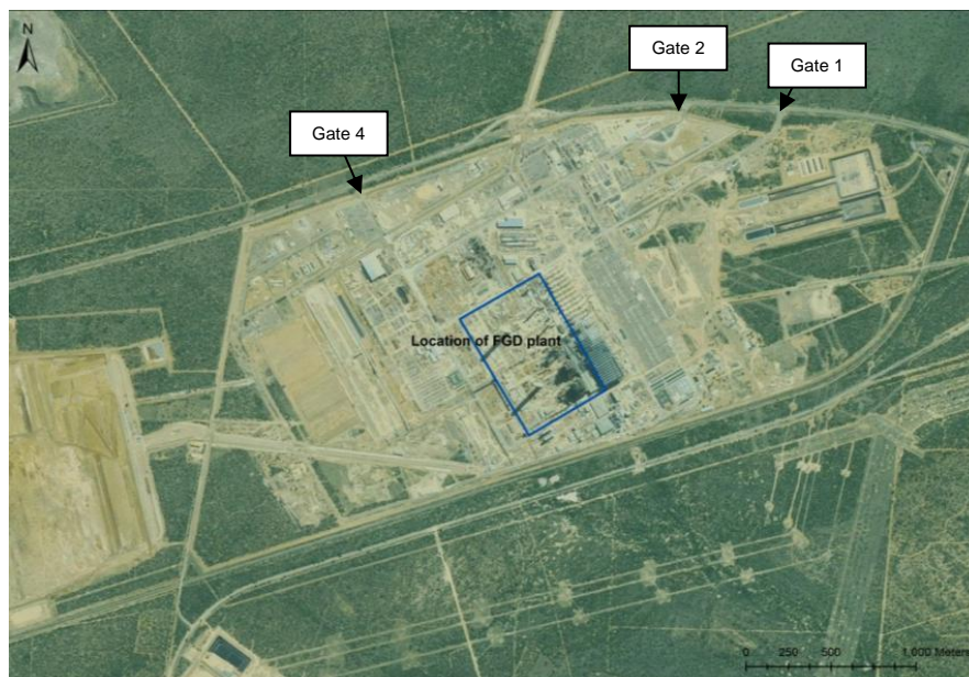
Figure 2.1: Location of FGD plant within Medupi Power Station
